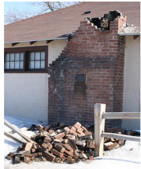
Chimney damaged by the 2008 Wells earthquake (Photo: Nevada Bureau of Mines and Geology Special Publication 36, 2011)
