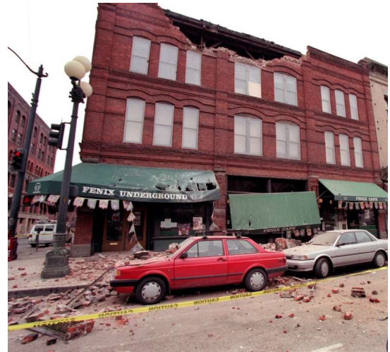
An unreinforced masonry building in Seattle damaged by the magnitude 6.8 Nisqually earthquake in 2001. (Photo: FEMA)
