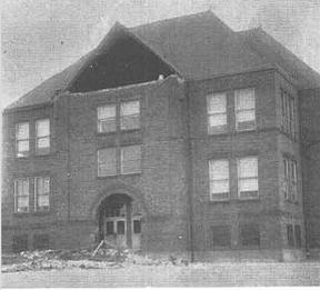
Above: Lafayette Elementary School in West Seattle was condemned and torn down due to damage from a M7.1 earthquake in 1949.
