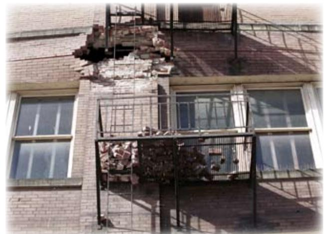
**The brick wall anchoring this fire escape failed during an earthquake, blocking this as a means of escape. Photo: FEMA**
