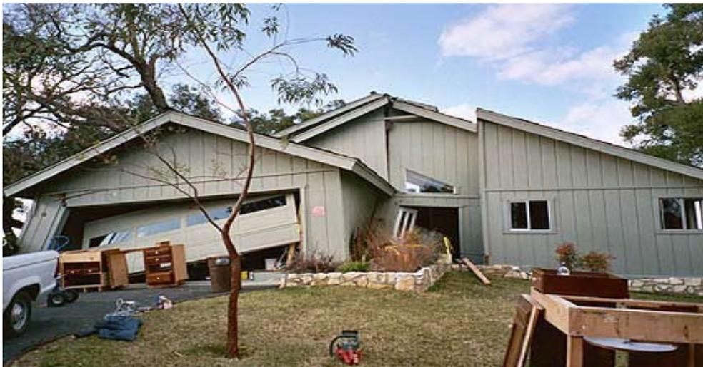
This house moved two feet off its foundation, breaking all utility lines, causing serious structural damage, and making it uninhabitable. Photo: FEMA
