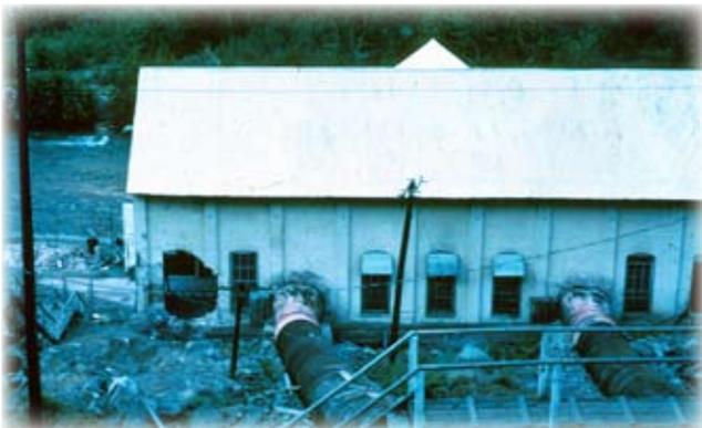
**This powerhouse on the Truckee River has a nine foot hole caused by a boulder falling into it after an earthquake. Landslides and rockfalls will be a substantial problem after a Cascadia earthquake. Photo: Federal Emergency Management Agency (FEMA)**
